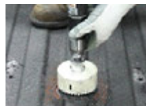
Use the pilot hole for error-free drilling
