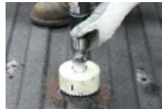
Use the pilot hole for error-free drilling
